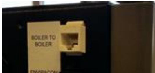
RJ45 Boiler to Boiler/EMS RJ45 Communication Port on Side of Boiler
